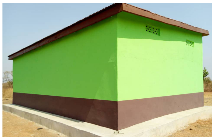
Warehouse constructed with gravel blocks in Fuu, Ghana.
